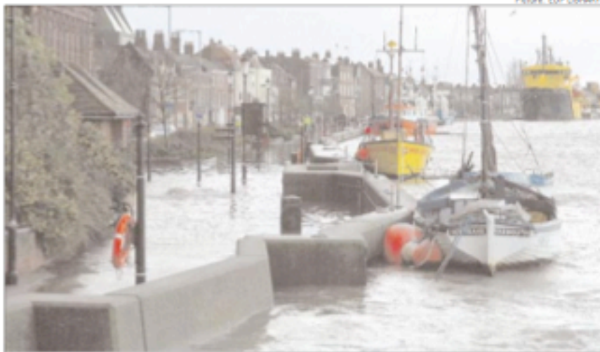
IN DANGER: Flooding in Yarmouth near the Haven Bridge last year.
